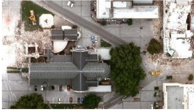
Figure 14 – RGB image of Christchurch post 2011 earthquake showing the extent of building damage
