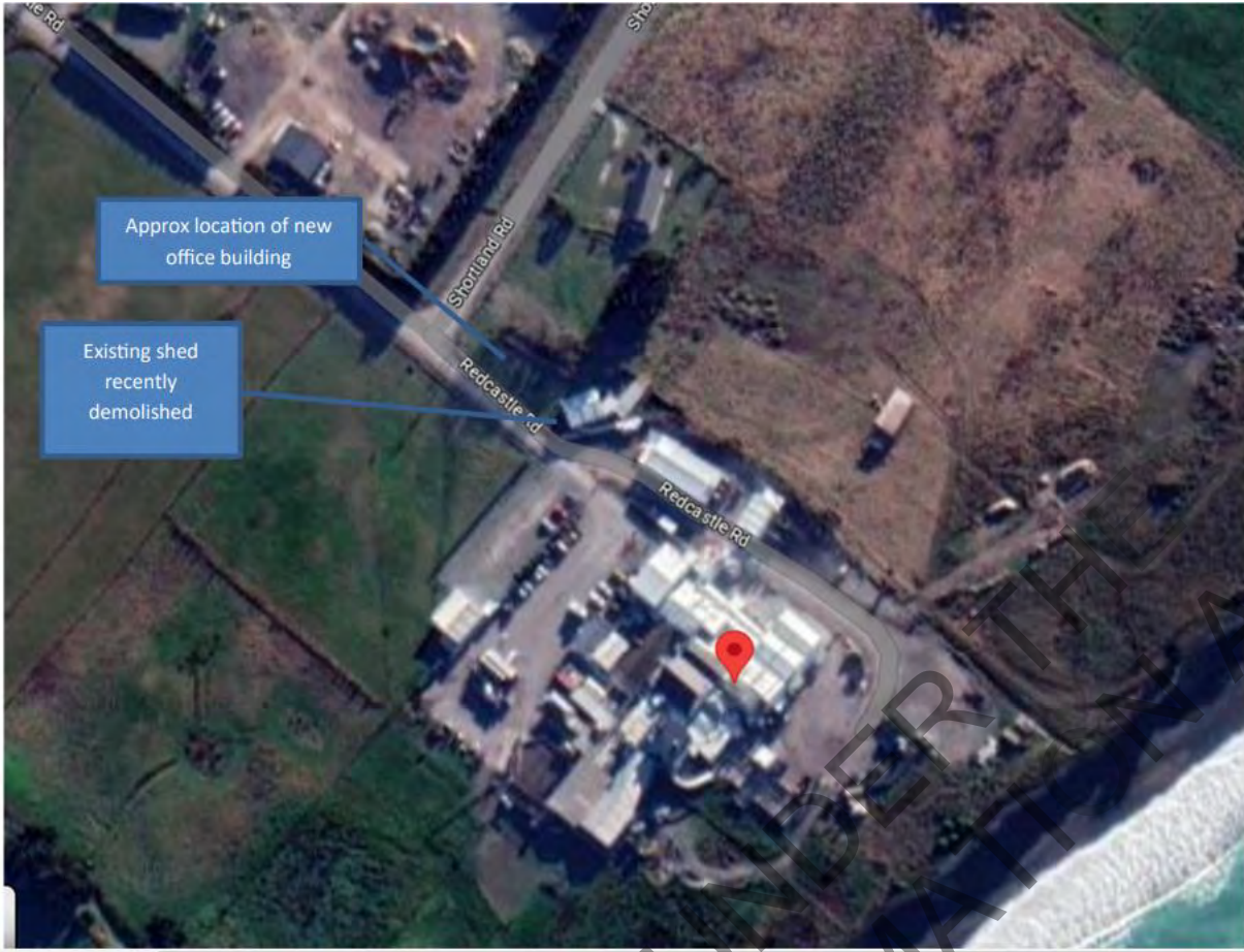
Figure 3. Aerial of site showing factory to south (red marker) source application.
