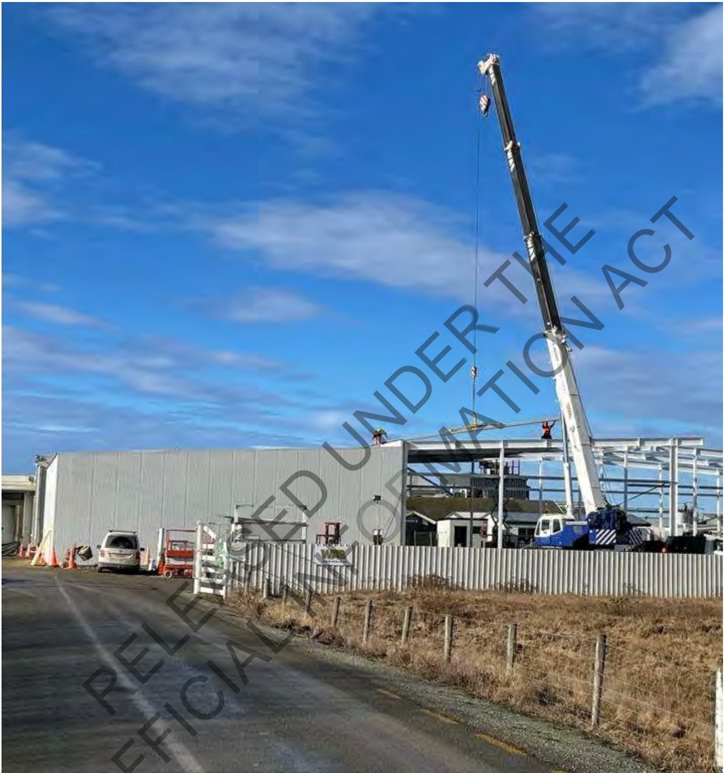
Blast freezer cabinets, capacity 60mt – insulation laid on the floor concrete to poured next week
