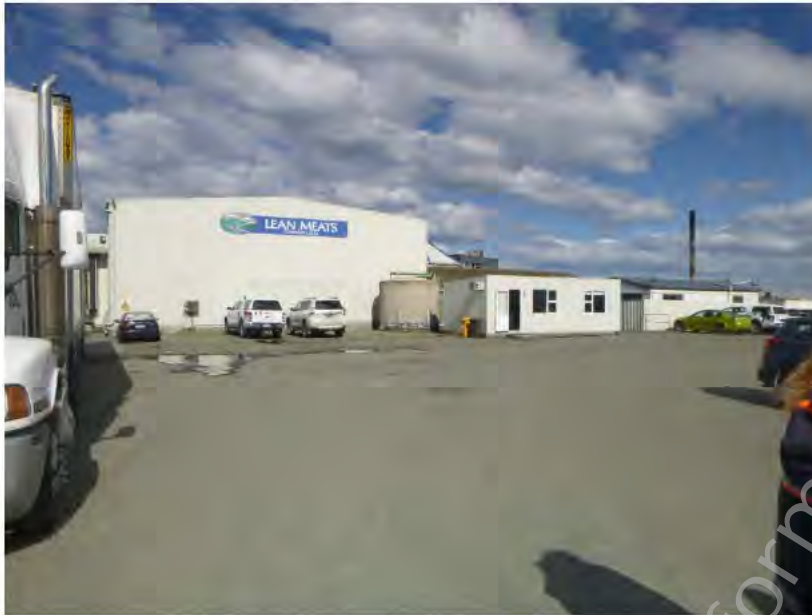
Figure 1: Entrance to NZ Binxi - Oamaru
