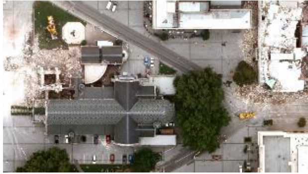
Figure 14 – RGB image of Christchurch post 2011 earthquake showing the extent of building damage
