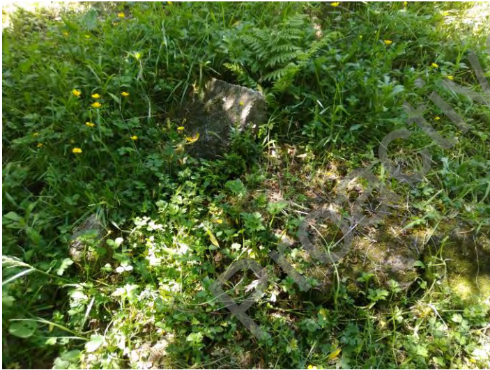
L5 – concrete/ceramic protrusion
