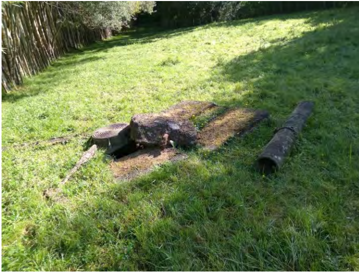
B1 – cement block/piping debris
