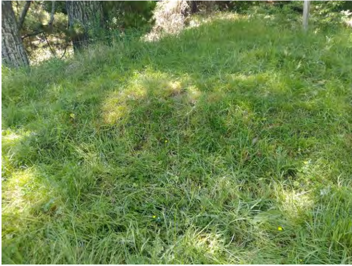
K6 – minor subsidence
