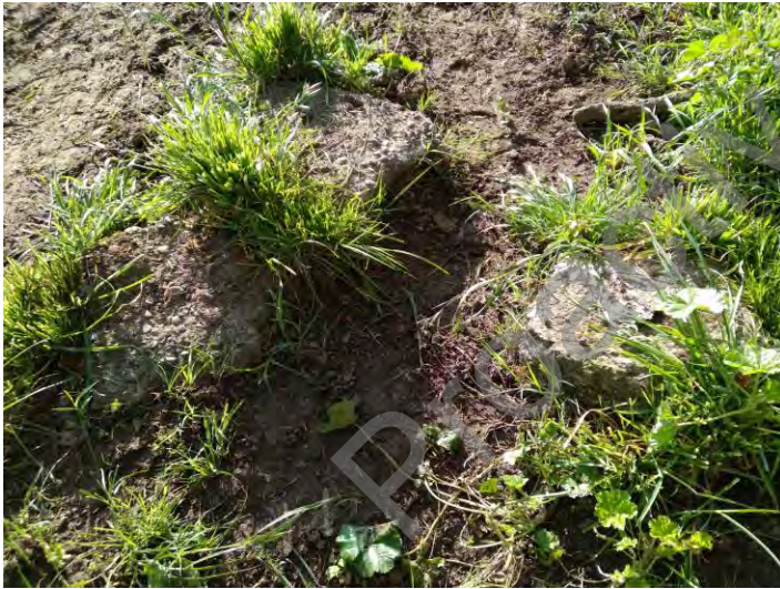
C7 – mixed cement blocks
