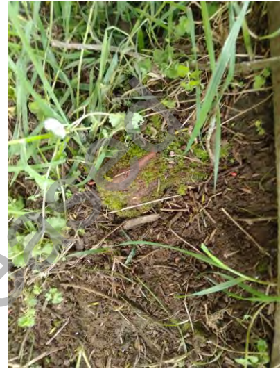
N6 – brick protruding
