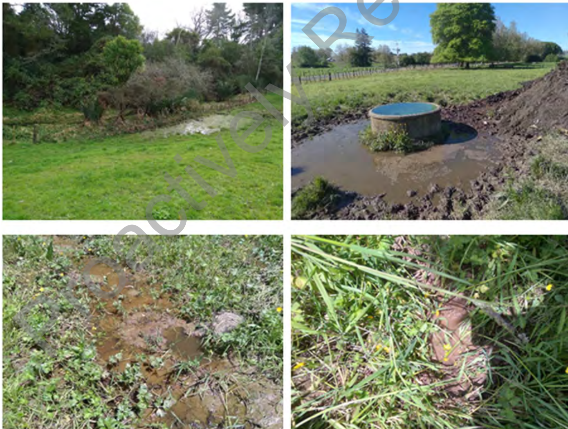
Figure 11: Areas of ponding observed across the landfill site (Top Left H4, Top right D7, Bottom Left K4, Bottom Right I7)
