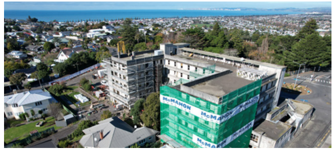
A drone image of the Hinepare Nurses' Home prior to demolition.
